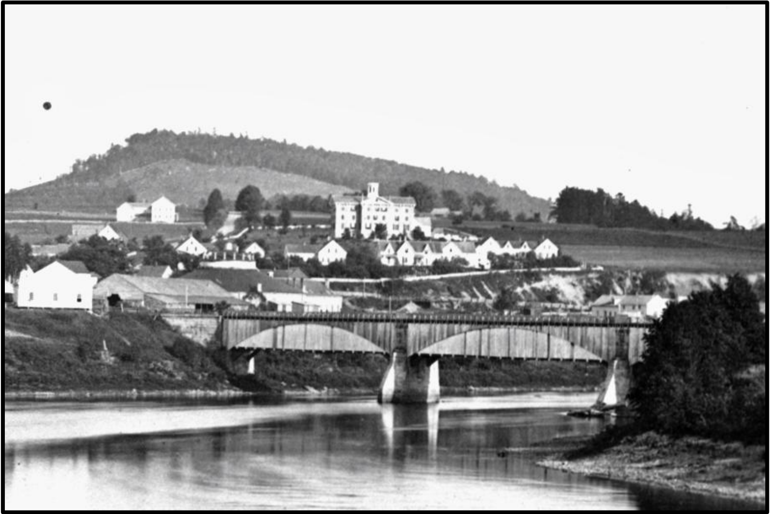
The first railroad bridge at West Lebanon - built spring 1848. Cost $21,600.; Three Spans at 200 Ft. = 600 Ft. Total Length. Image made in 1859.
