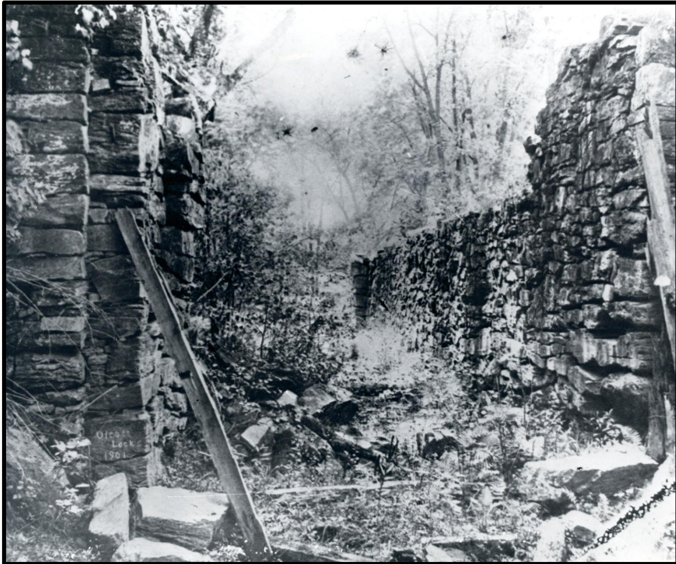
Remains of the Canal Locks at the Lower Falls in 1901 Each lock measured about 16' wide X 88' long
