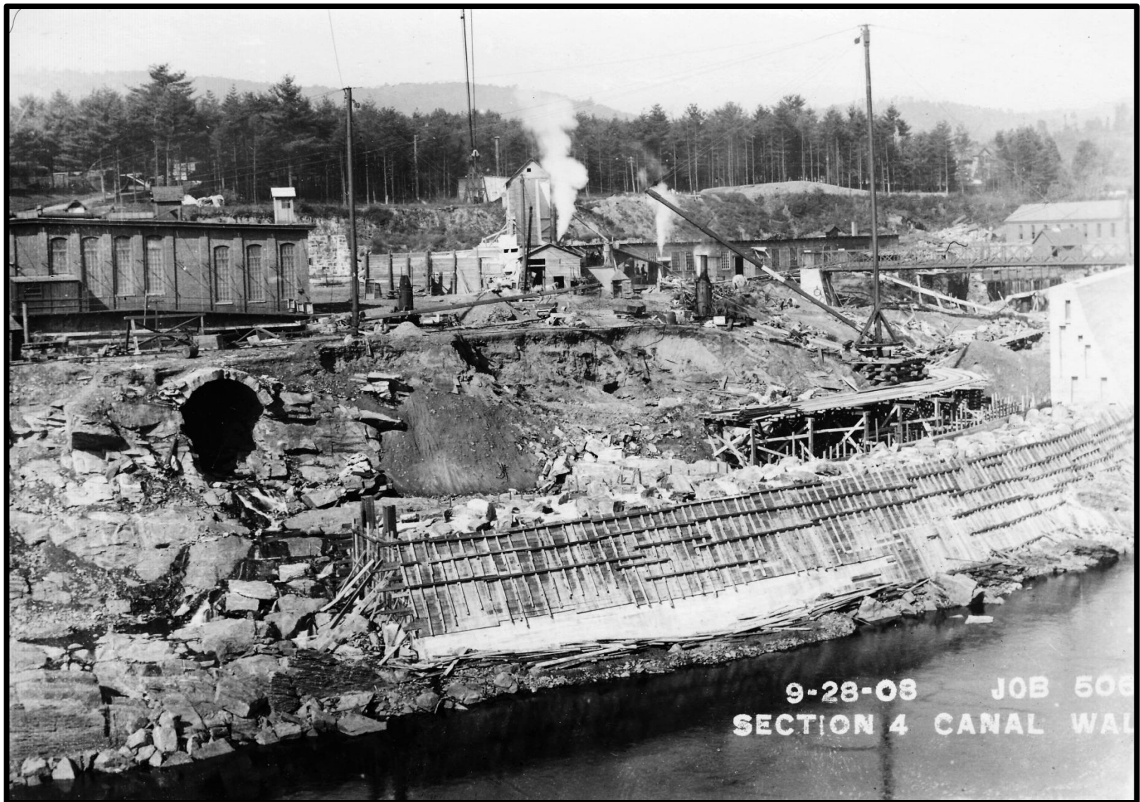
1908 new reinforced concrete canal wall under construction and preparing to construct the new electrical generating power house
