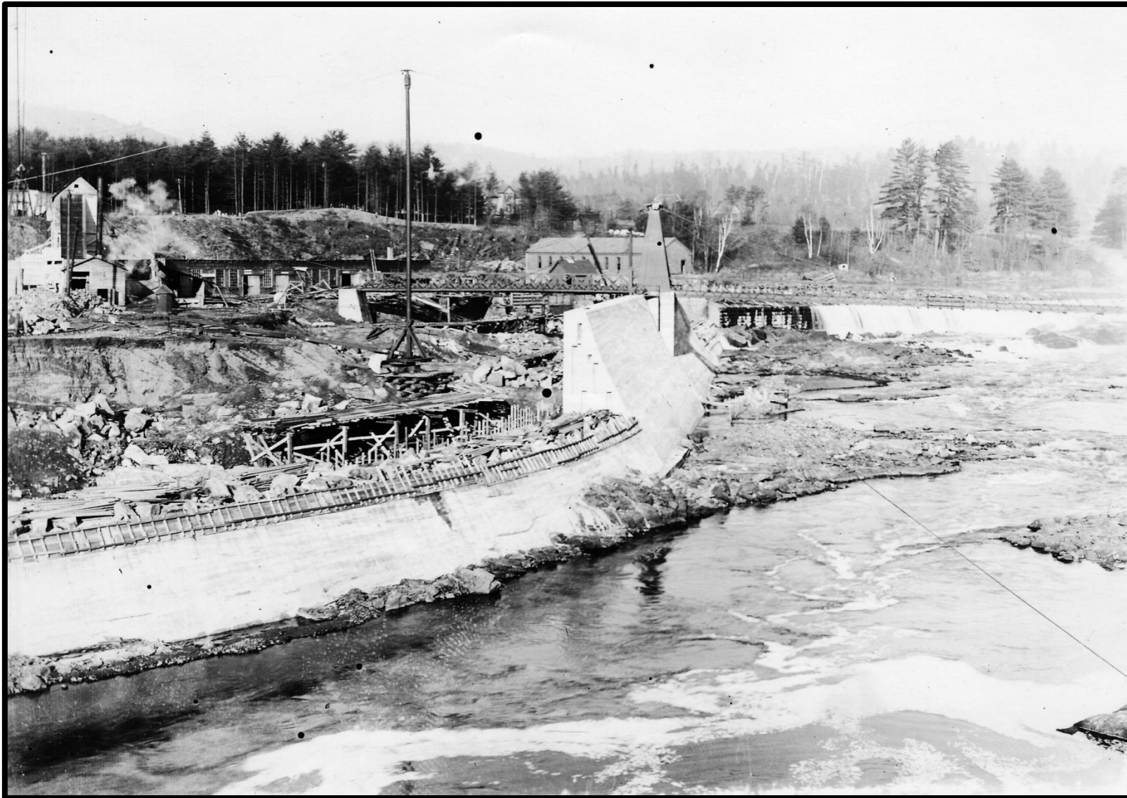
In 1908 the original dam and canal works constructed of wood and rock was replaced by poured in place concrete. View of the canal wall under construction.
