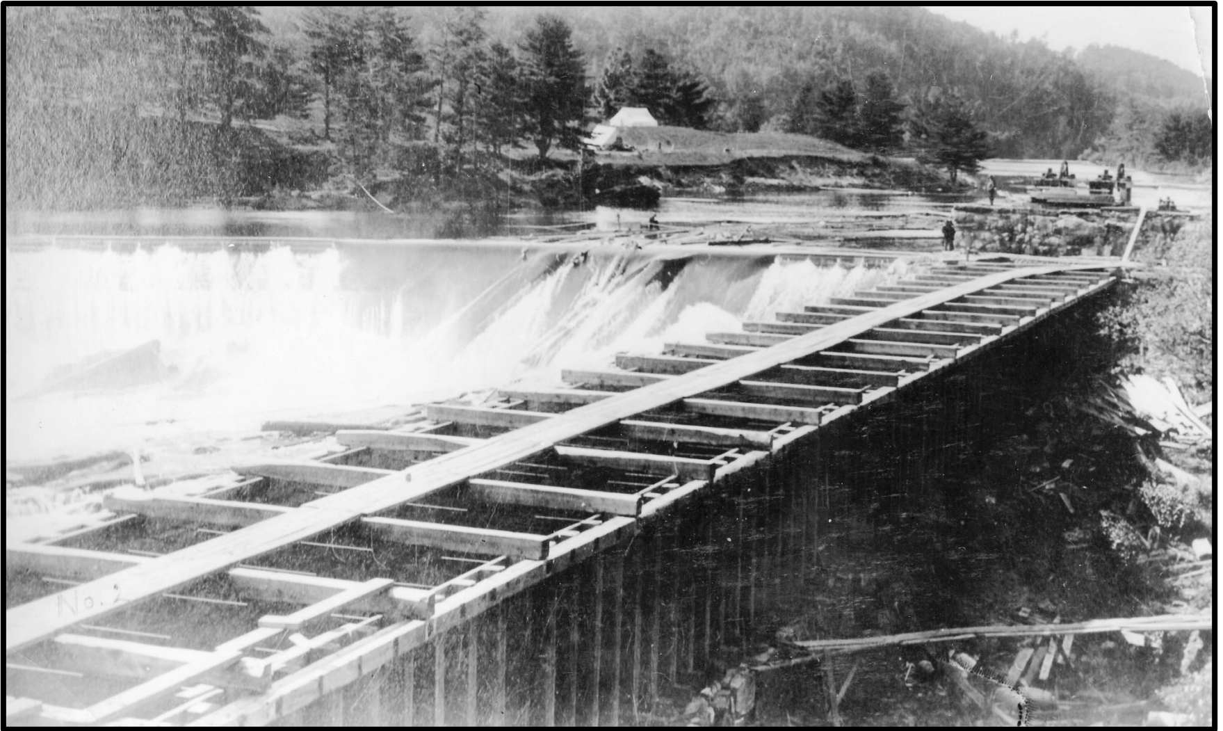
The wooden canal that fed water to the new pulp grinding building constructed in 1890. 10 grinders developing 2,250 hp each.
