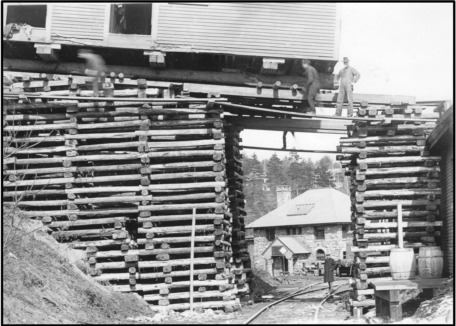
Moving a building within the paper mill complex. In the background is the company's stone office building.
