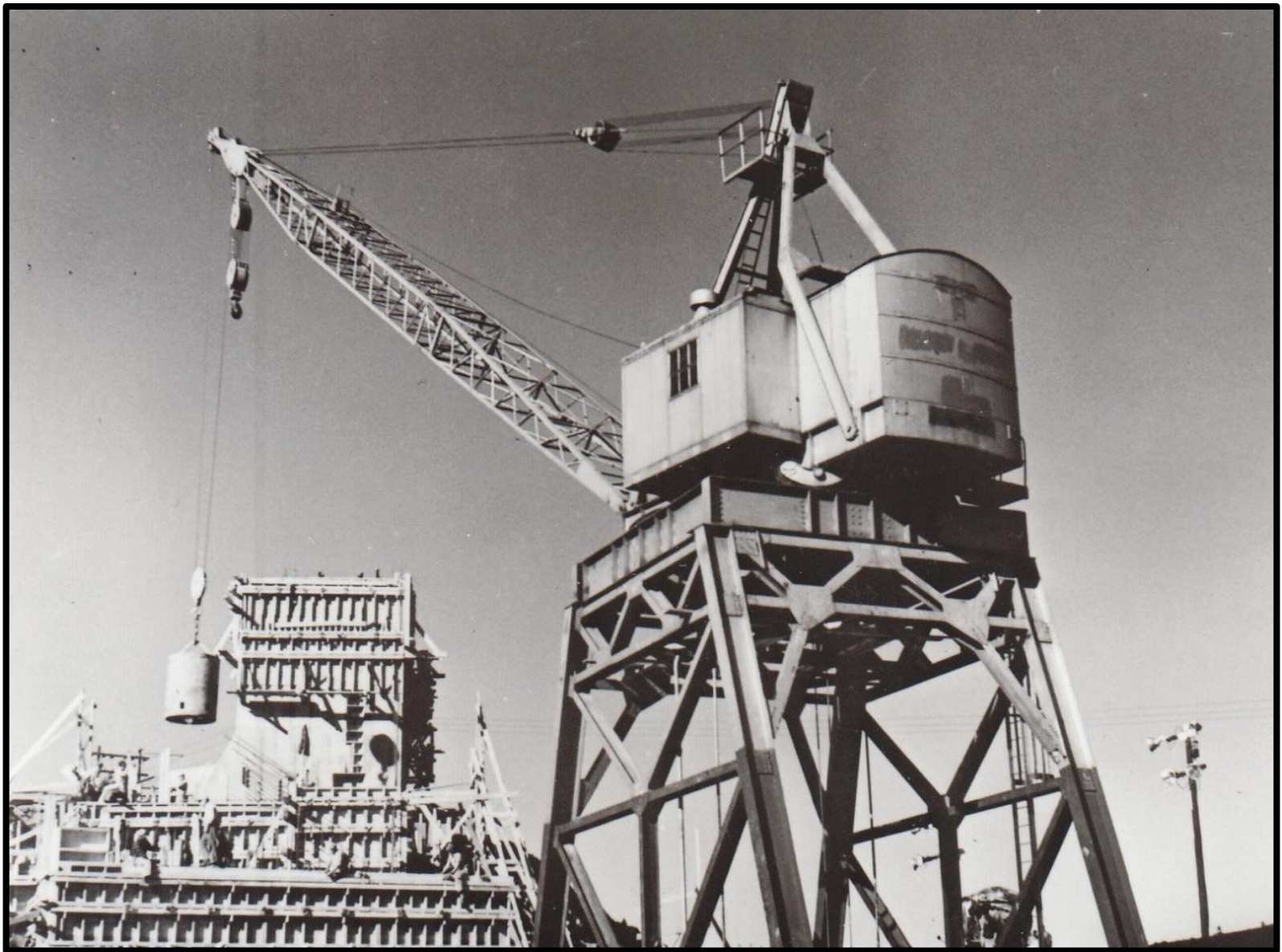
Construction of Wilder Dam. Pouring Concrete.
