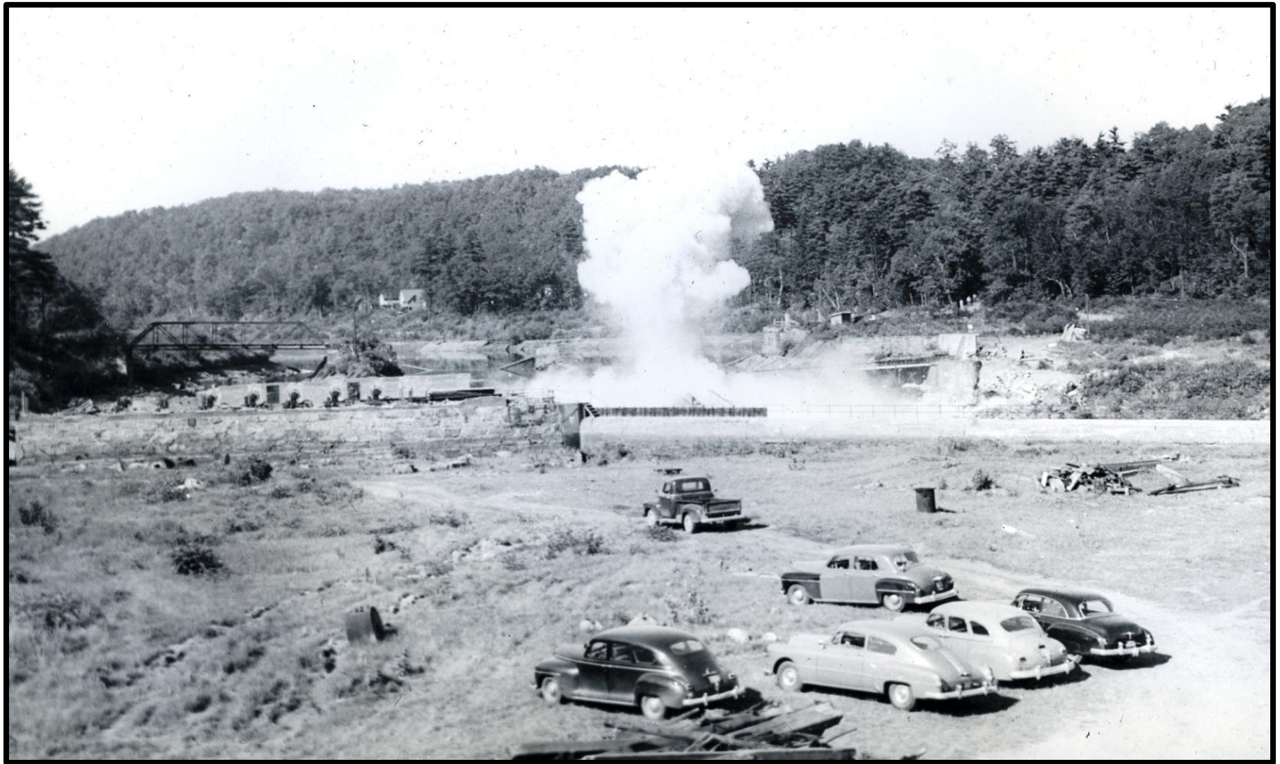
Dynamiting the old paper mill dam. Looking upstream 1950
