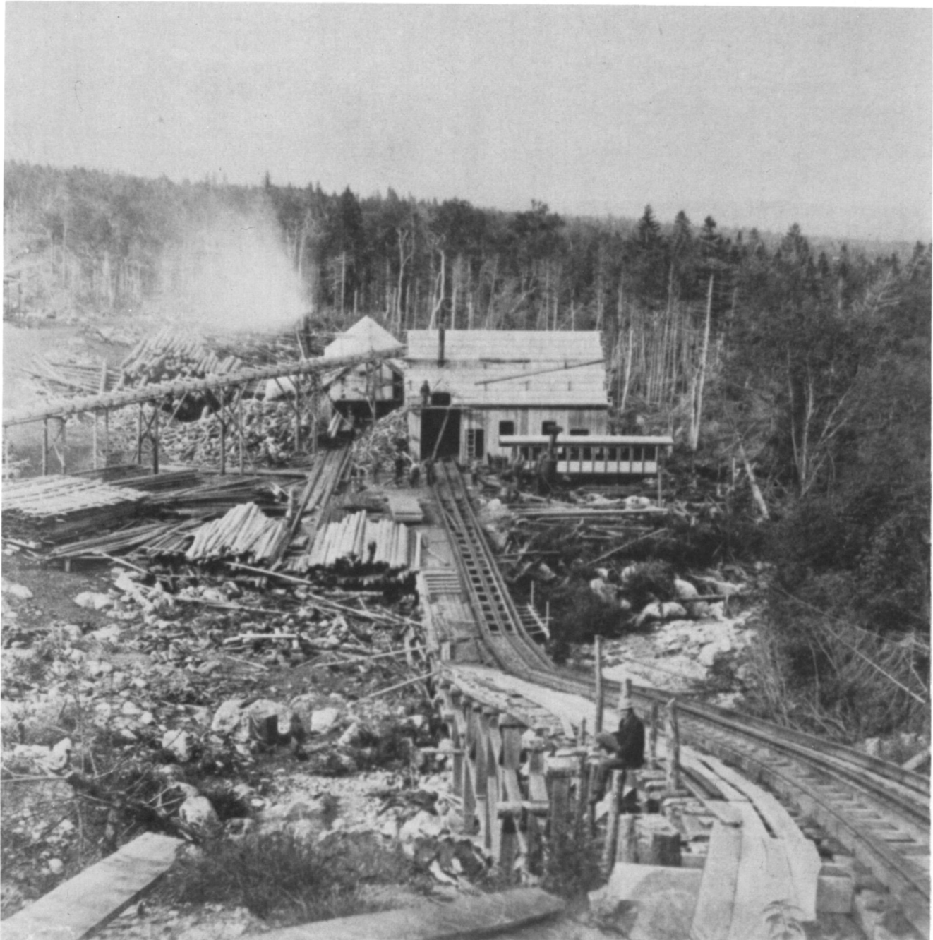
Figure 6. A scene at the base of the Cog Railway during early construction, c1867–68. Old Peppersass and the early “closed” coach are alongside the newly constructed enginehouse and shops. There is a sawmill in the background, and a viaduct (left) is carrying water from Ammonoosuc Brook to the mill and railway. Courtesy of the New Hampshire Historical Society, stereograph S11.
