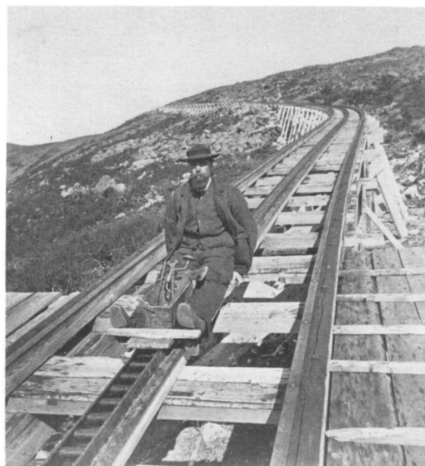
Figure 16. A workman descending Jacob's Ladder on a slideboard, or "Devil's Shingle," c1870. Note the toolbox sitting in front, between the workman's feet. The original strap-iron rails were still in use, and the platform used at Jacob's Ladder for unloading and loading passengers is visible at the right. Courtesy of the New Hampshire Historical Society, stereograph S5.
