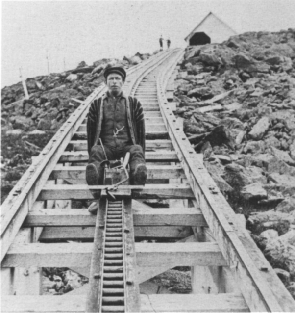
Figure 17. A workman about to leave the summit of Mount Washington on a slideboard for a trip down the railway, c1870–71. The newly built enginehouse-depot is visible at the rear. Courtesy of the New Hampshire Historical Society, stereograph S19.
