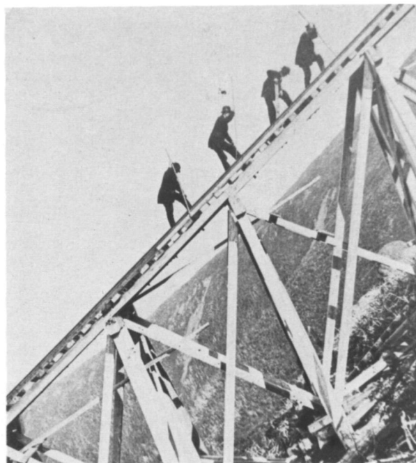
Figure 12. An early view of Jacob's Ladder, the highest and steepest trestle on the Cog Railway, inclined at a grade of 37.41 percent, 300 feet long, and rising to a maximum height of 25 feet above the ground. The caption reads "Jordan am a hard road." Courtesy of the New Hampshire Historical Society, stereograph S35.
