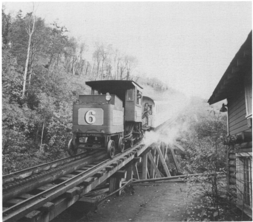
Figure 24. Cog Railway locomotive #6 (Great Gulf) arriving at the Base Station, 1994. The locomotive precedes its "closed" coach into the station, slowing its descent as it "lowers" the coach into the station. Photo by the author.
