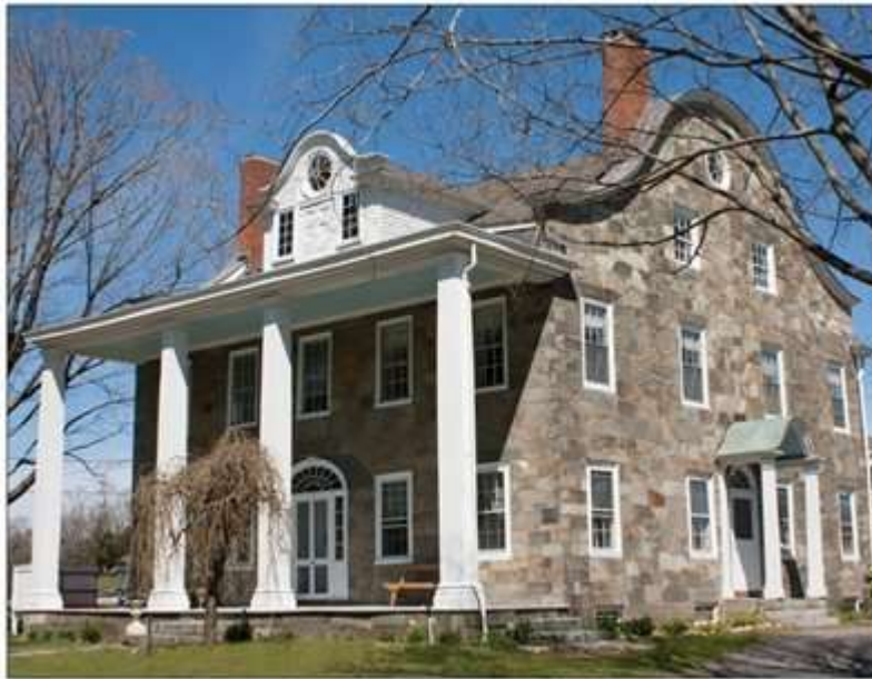
Hearthside House, built ca 1810
