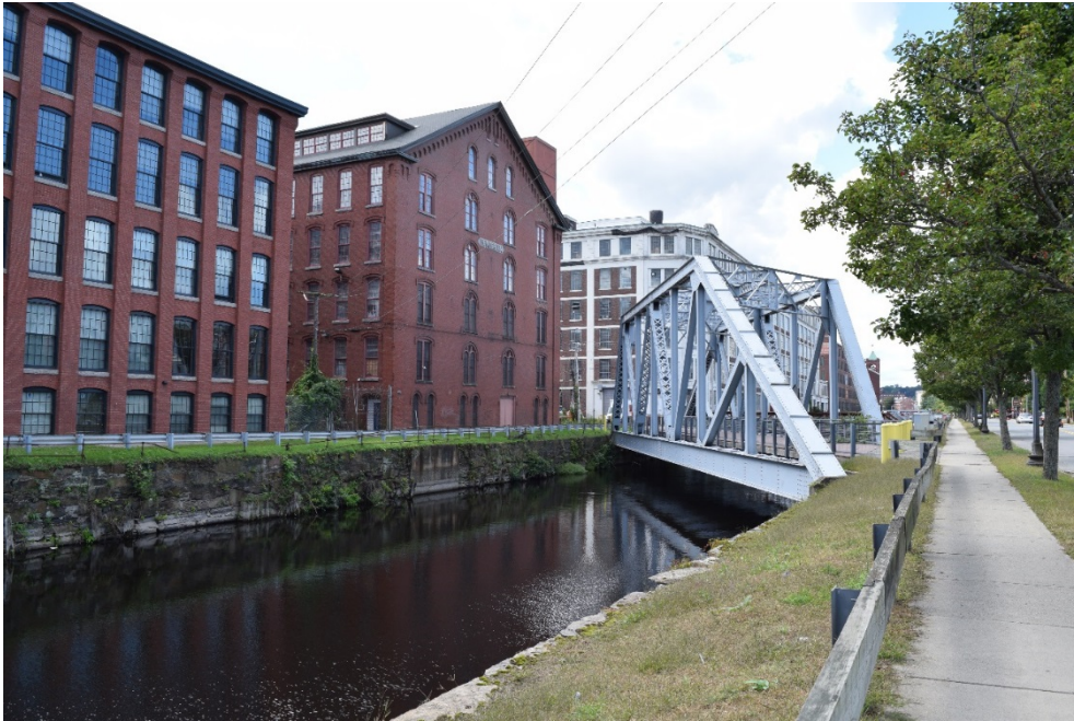
Lawrence Duck Co. mill, Pemberton mill, and American Woolen Co. mill along North Canal, Lawrence, Mass.
