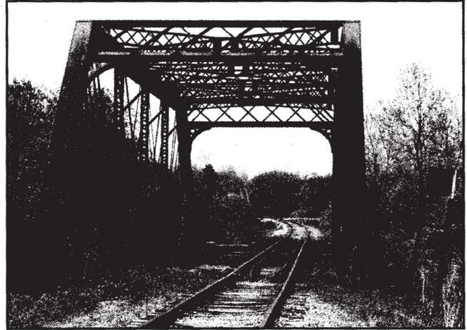
*Two views of the Atlantic & St. Lawrence Railroad's steel through-truss bridge spanning the Royal River in Yarmouth, Maine. In the photo on the left, note the space on the left once occupied by a second track.. Nelson Lawry photo.*
