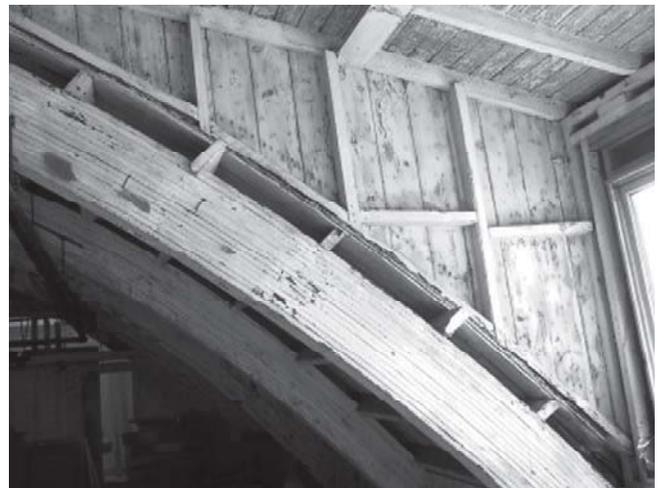
*Arch formed with 15 nailed laminations of one-inch thick (nominal) lumber.
