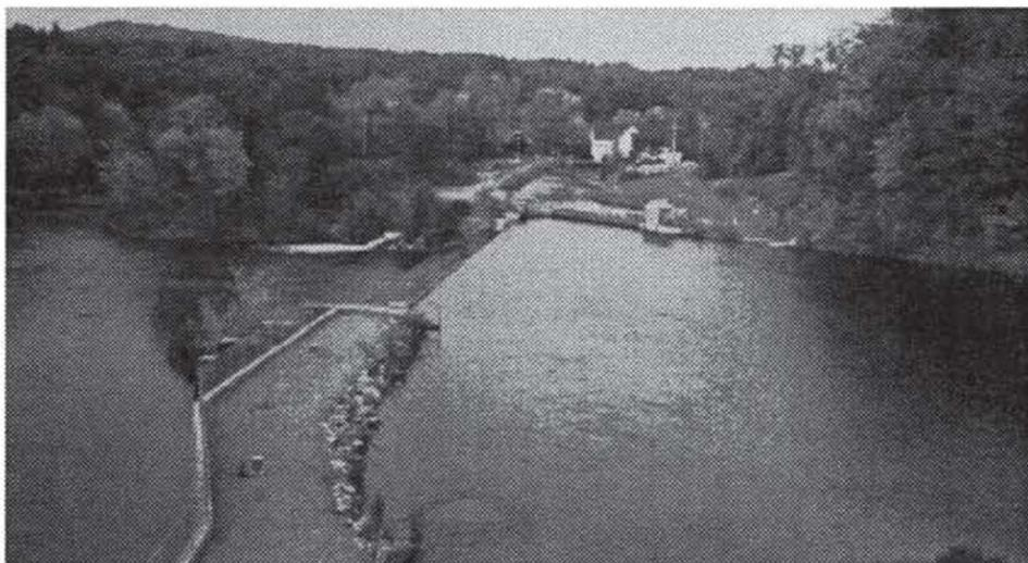
*A view downstream from the top of the Hopkinton flood-control dam where a second, hydropower dam is seen. A canal supplying the hydroelectric generation station is in the distance, beyond the spillway.*
