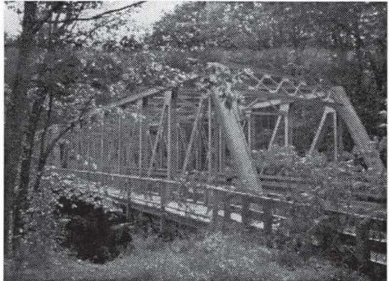
*This two-span riveted Pratt truss bridge, also attributed to John Storrs, was erected in 1933.*
