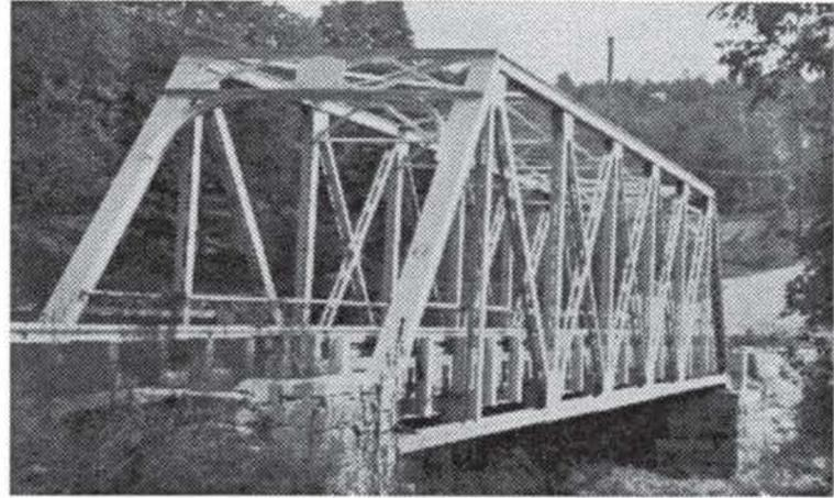
*One of two riveted Pratt truss bridges crossing the Contoocook River in West Henniker near the industrial complex remains visited during the NNEC Fall tour. Erected in 1915, the bridge was designed by New Hampshire's first State Engineer, John Storrs. It rests on dry laid stone abutments, which have recently been strengthened with concrete pads.*
