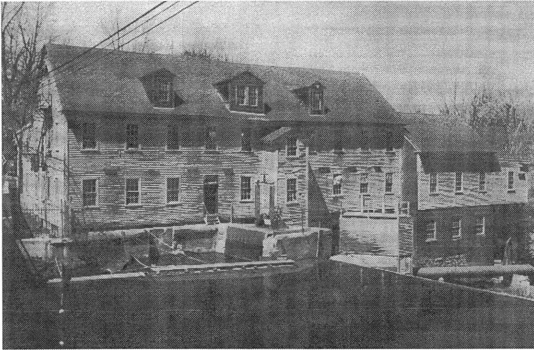
*Fig. 3 The Burleigh woolen mill was constructed during the 1850s at Rocky Gorge, South Berwick, ME, using the falls of the Great Works or Asbenbedic River for the essential waterpower. The main mill building shown is a unique clapboard-over-brick construction. The Great Works mill site is one of the oldest in Maine, in use since the mid- 17th century.*
