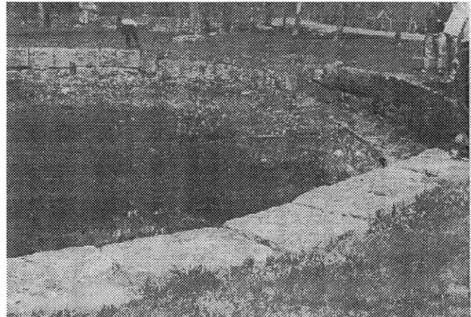
*Fig. 2. The granite-block turntable pit and foundation beyond it for the threebay locomotive house, were built for the Portsmouth, Great Falls & Conway Railroad at Conway Junction, South Berwick, ME. The junction was later renamed Jewett by the Boston & Maine Railroad.*
