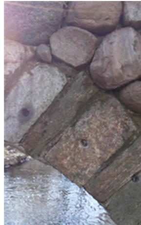
Stone arch dike features, including voussoirs (left) and uncoursed, dry-laid, rounded stones supported by stone masonry walls (right)
