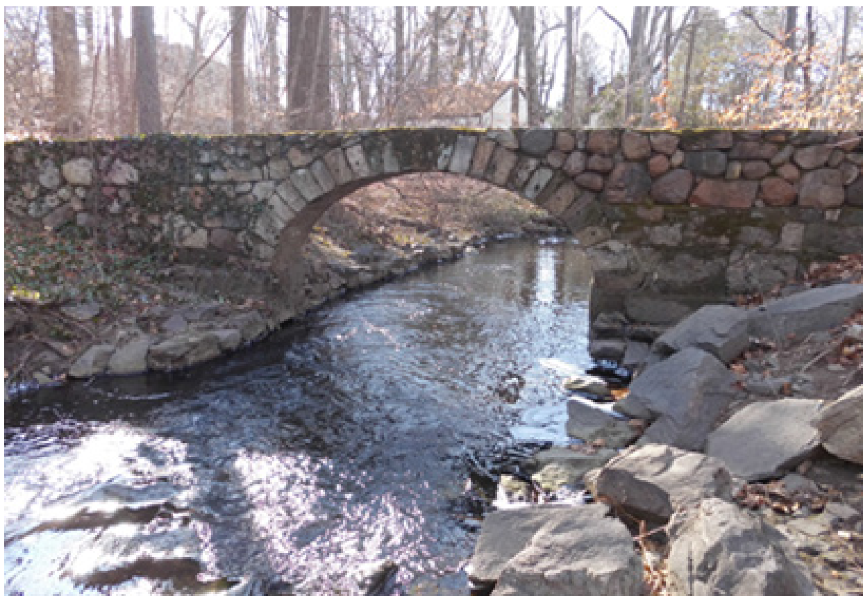
Upstream fascia of stone arch dike along Greenwich Creek
