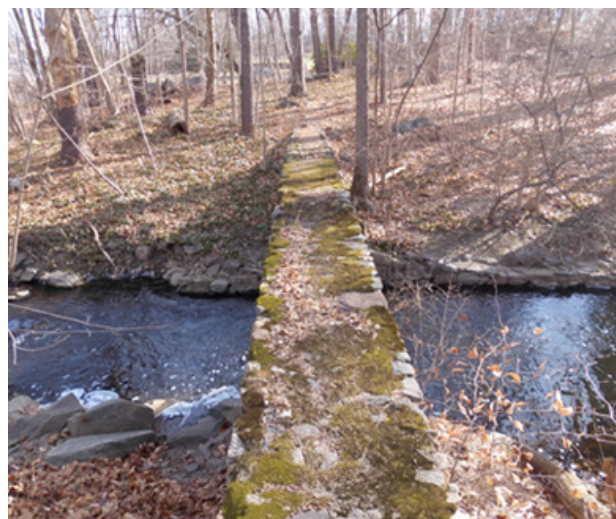
Top view of stone arch dike along Greenwich Creek from west approach
