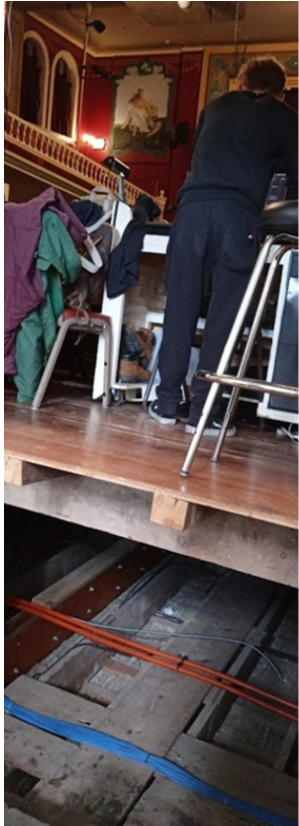
Under the Opera House's movable floor
