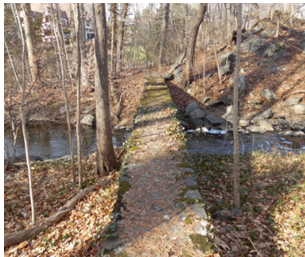
Top view of stone arch dike along Greenwich Creek from east approach
