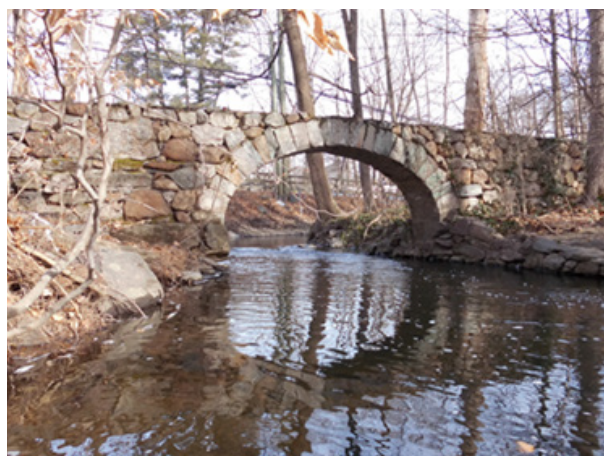
Downstream fascia of stone arch dike along Greenwich Creek
