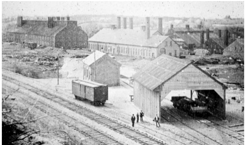
Undated photo of the ironworks
