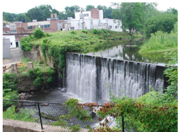
Looking at the dam with the plant in the background c. 2020. (No attribution)
