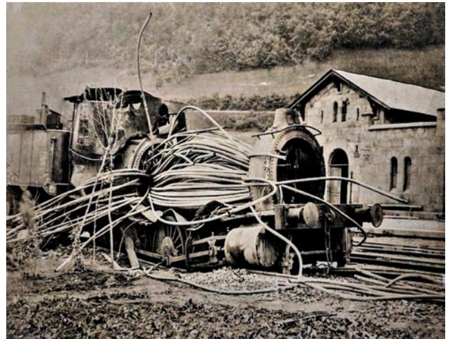
Fig 2 Boiler explosion, Germany. The consequence of a faulty safety valve? Many Trade journals would dedicate an entire page to boiler explosions. (google)
