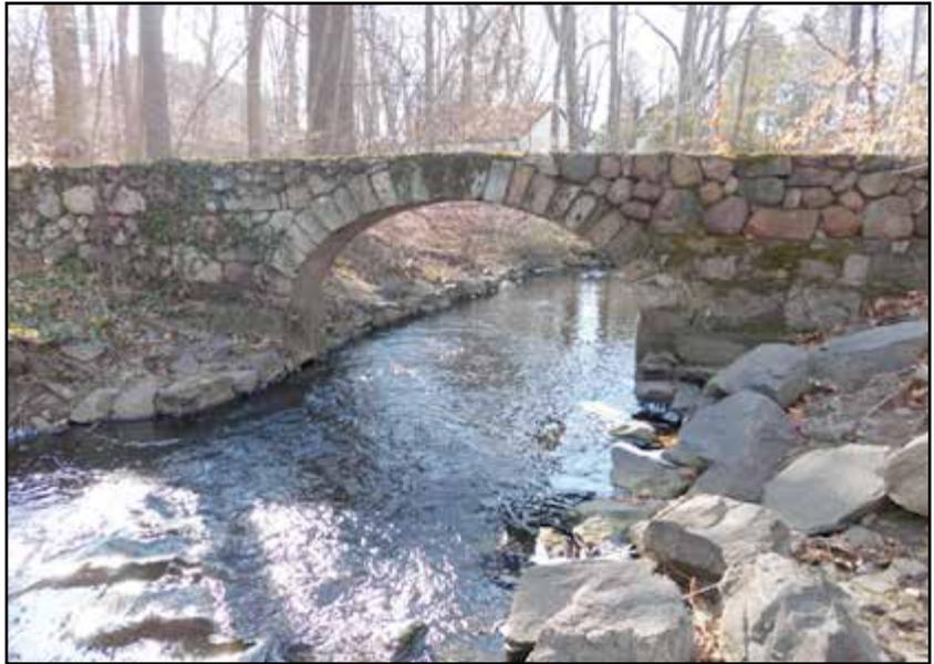
Figure 1. *Upstream fascia of stone arch dike along Greenwich Creek.*
