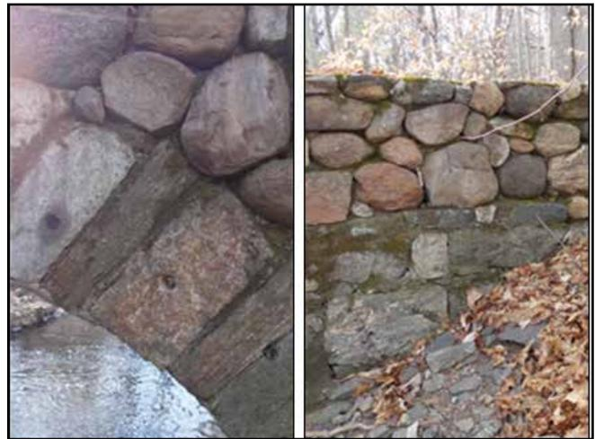
Figure 5. *Stone arch dike features, including voussoirs (left) and uncoursed, dry-laid, rounded stones supported by stone masonry walls (right).*
