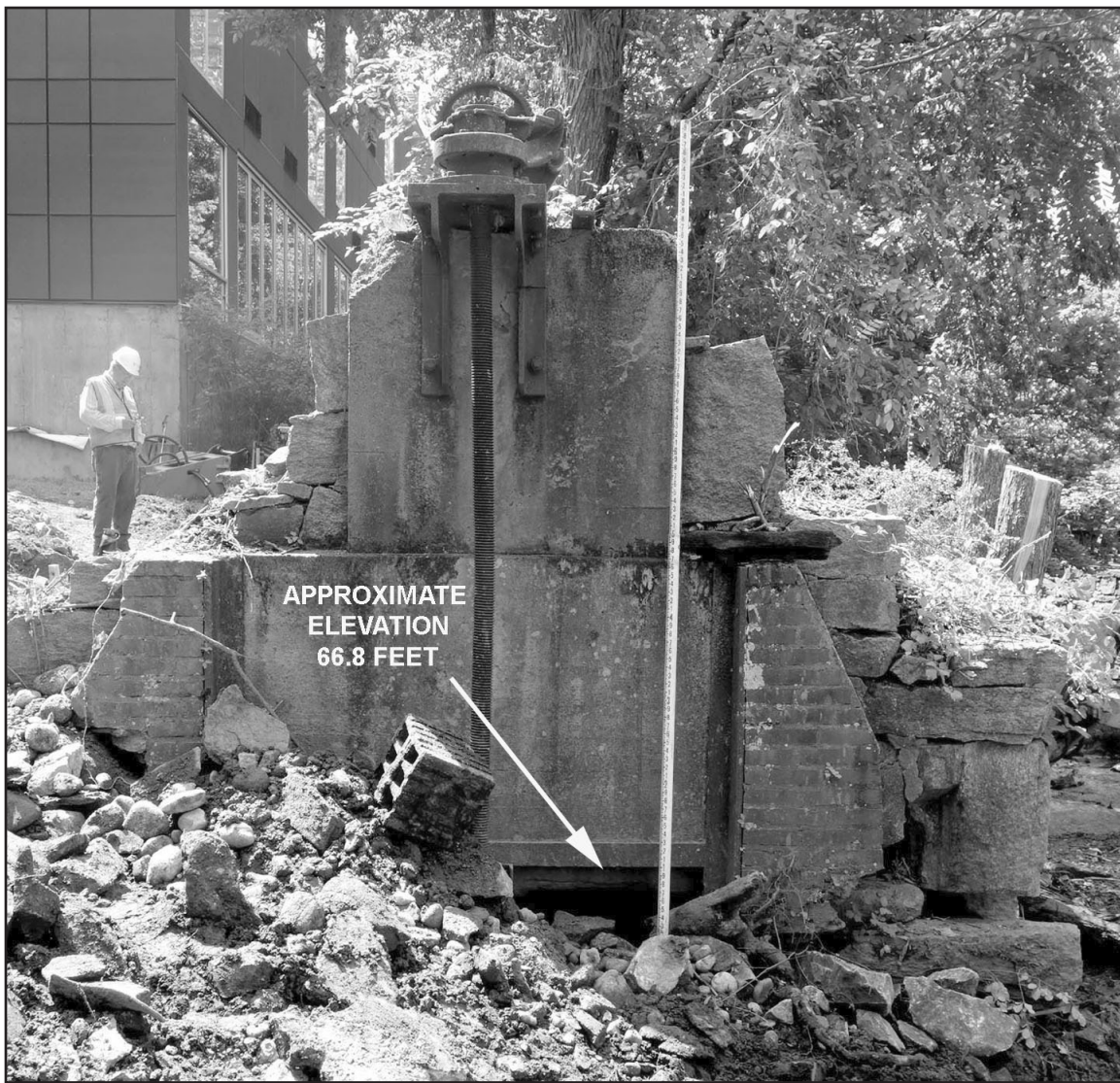
Figure 9. 2018 view south of sluice gate exposed after dam demolition.
