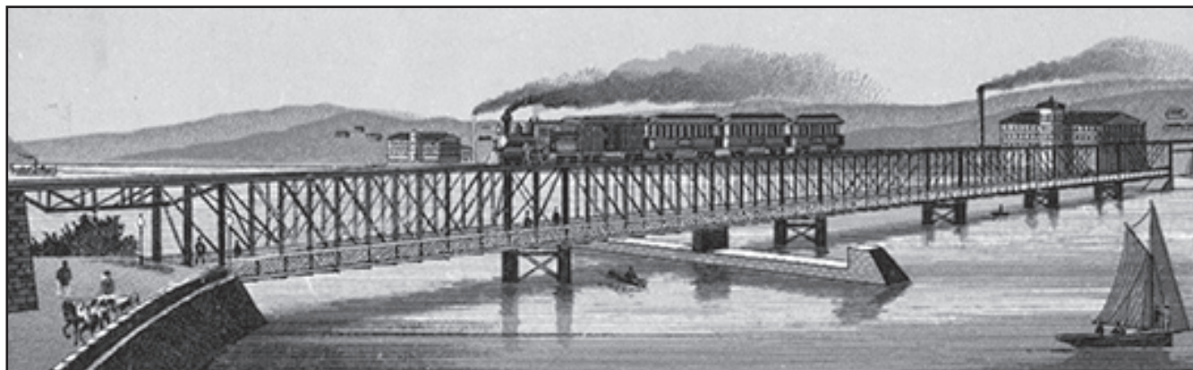
An early depiction of the Slade's Ferry Bridge across the Taunton River between Fall River and Somerset, Massachusetts. Rail traffic crossed on the upper deck, while vehicular and pedestrian traffic used the lower deck. This view shows how the roadway split on the Somerset side. A similar split occurred on the Fall River side, in the vicinity of Mechanics Mill.
