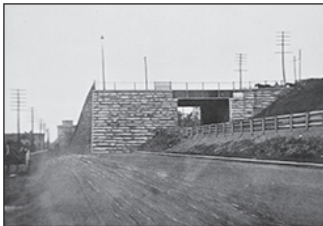
1906 view of the "Davol Street Ramp", one of the more unusual features of the Grade Elimination Project. It carried Walnut Street over the tracks with a sharp bend and ramp down to Davol Street.
