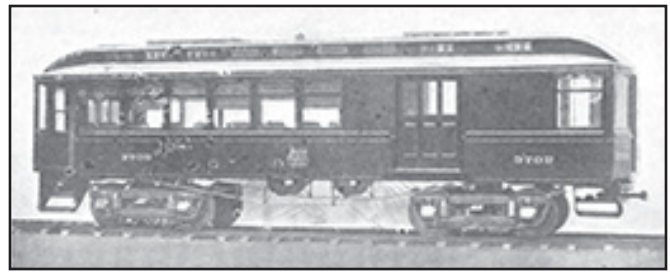
A Brill combination passenger and baggage car used by the New York, New Haven and Hartford Railroad on the Providence to Fall River route, from Street Railway Journal, March 1902.
