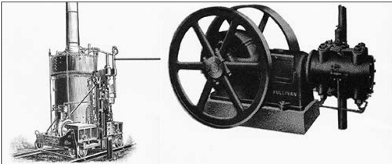
*Sullivan rock channelers (left) were used to drill patterns of deep holes to split rock without using explosives. Sullivan air compressors (right) were widely used in mining and road building also.*
