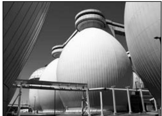
*Fig. 4. Walking amongst the digesters. Each is about 90 feet in diameter and 130 feet tall made of boiler steel. Most were built by the Chicago Bridge & Iron Co.*
