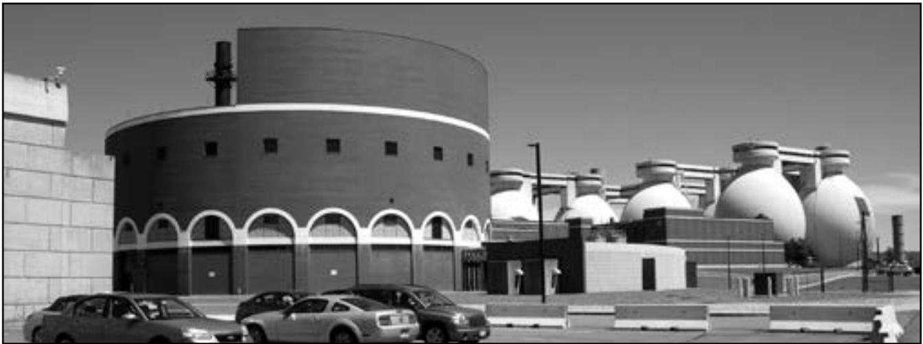
*Fig. 2. The round brick building is the South System Pump Station; beyond it are odor control and centrifuge buildings and egg-shaped digesters rising in the distance.*
