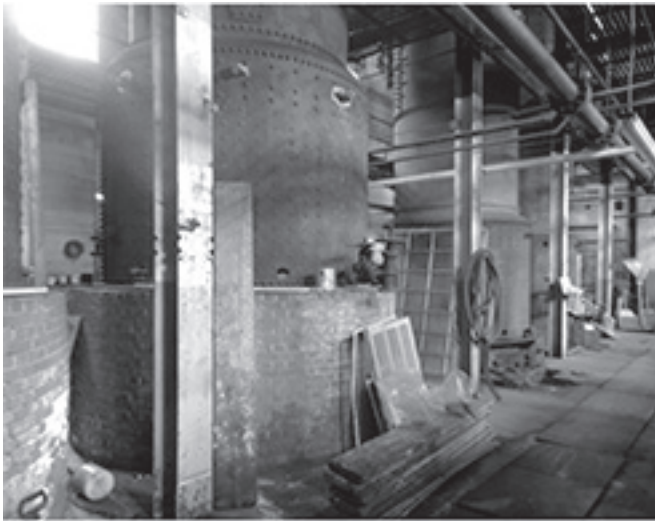
View of the four remaining 300-hp Bigelow-Manning upright boilers. One of the two newer Babcock & Wilcox boilers is visible in the distance. The plant also contains two Cleaver-Brooks oil-fired units that are still in use by JA Manufacturing to provide heat and steam to its plant across the street.
