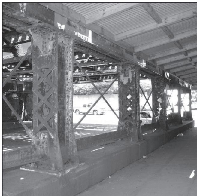
One of two trestle structures between the roadway and the sidewalks that form intermediate supports for the bridge.
