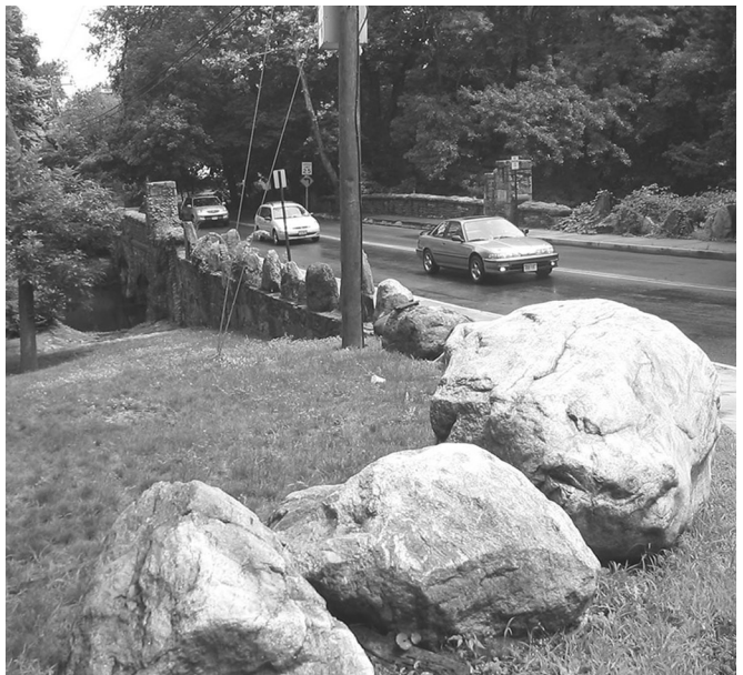
View southeast of Cold Spring Road Bridge border stones at northwest approach corner, with wingwall in background; larger boulders in foreground replaced original smaller upright stones similar to those on wingwall.
