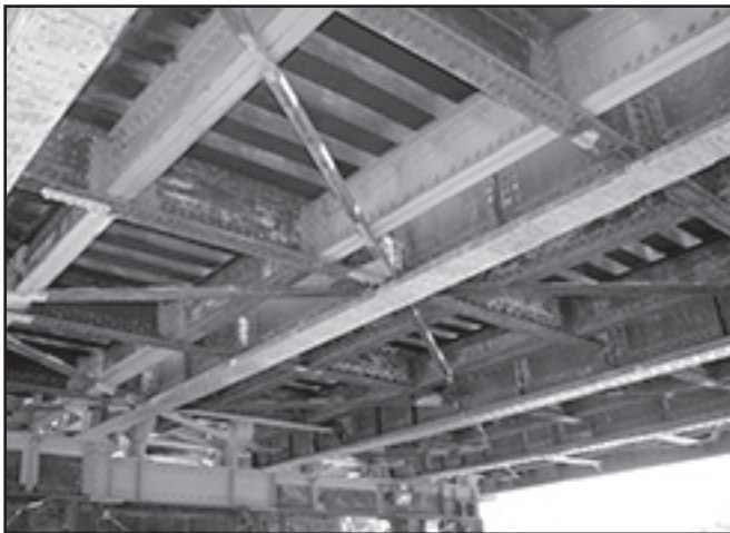
Underside, showing main girders, plate-girder floor beams, longitudinal stringers under the rails, and angle cross-bracing.
