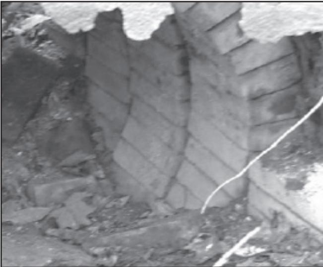
*Detail of the fire brick lining of the Taylor electric furnace.
