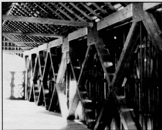
4. Interior view, 1975, showing the steel reinforcement plates added in 1974 ( National Register nomination photograph by D. Clouette ).
