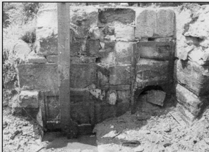
View West of Partially-Excavated Intake Structure Gate Frame Façade, After Removal of East Façade, with North Training Wall at Right, Lower Intake at Left with Immovable 1986 Gate That Served Sawmill Turbine
