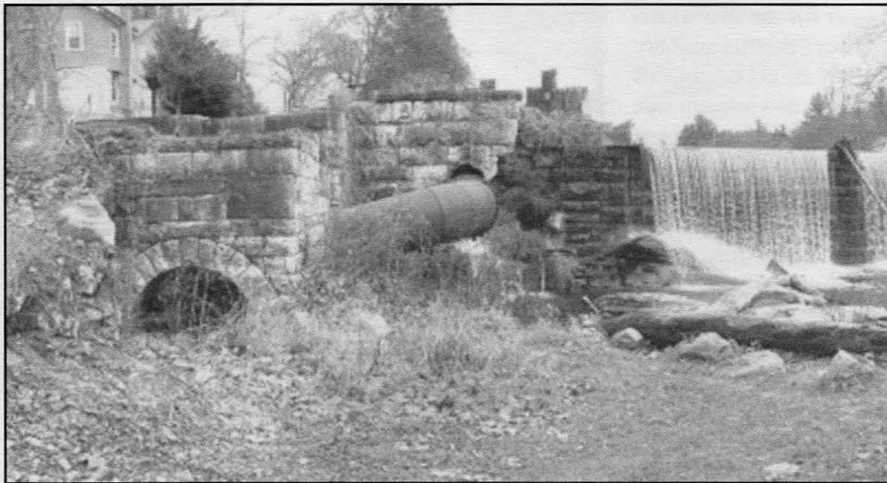
Left: View East of Wheelpit and Tailrace Arch (Left). Intake Structure with Penstock for Blowing Engine and Lower Pipe for Removed Penstock to Sawmill (Center), and North End of Spillway (Right)
