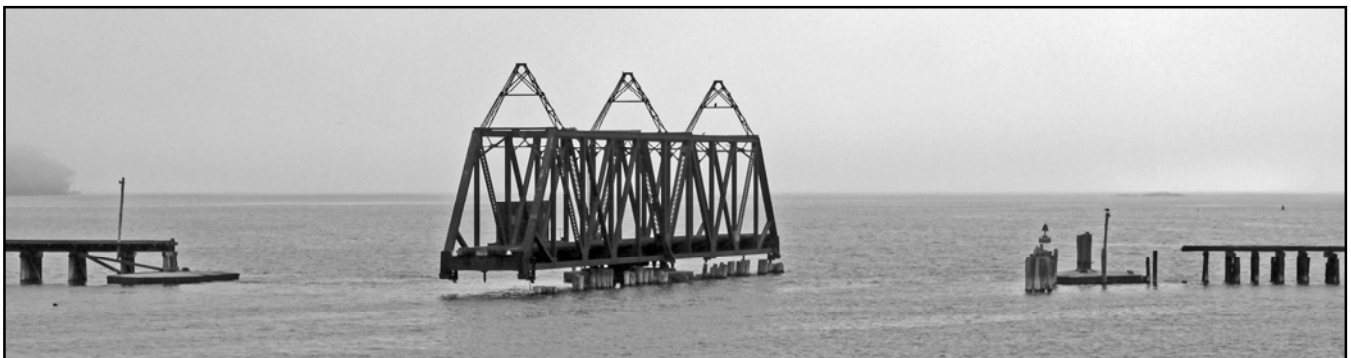
The Grand Trunk Railroad built a long timber pile bridge, with a central steel swing span, to carry its trains across the mouth of Back Cove to its station on India Street on the Portland waterfront. Part of the bridge suffered serious damage from fire in 1984, and has been out of service since then. Nelson Lawry photo.
