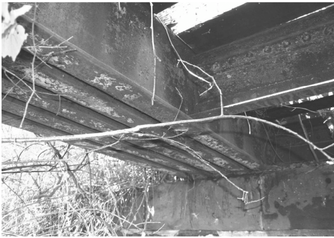
Detail of “5-ply” I-beam cattle-pass bridge, 1915, railroad-built using salvaged and new steel.
