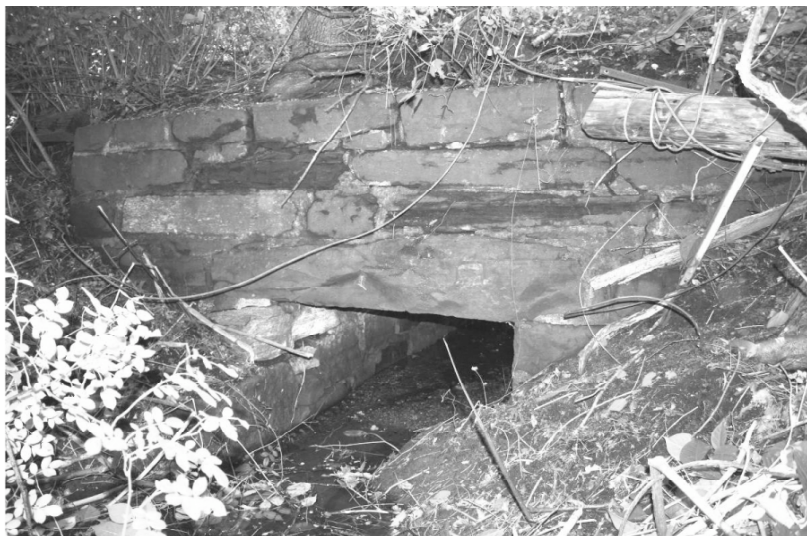
Simple stone box culvert on the former Canal Line in Simsbury, CT, possibly part of the line's original 1847 construction.
