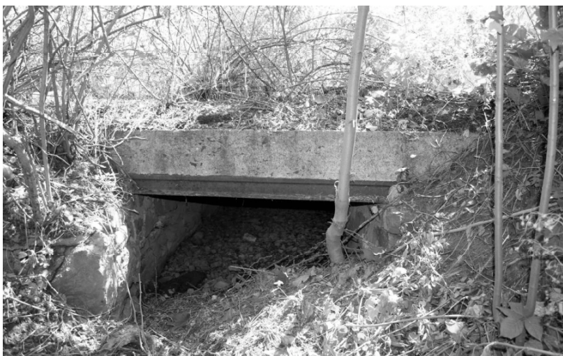
Rail-stringer and concrete-slab culvert, a ca. 1916 replacement for an earlier stone box culvert.
