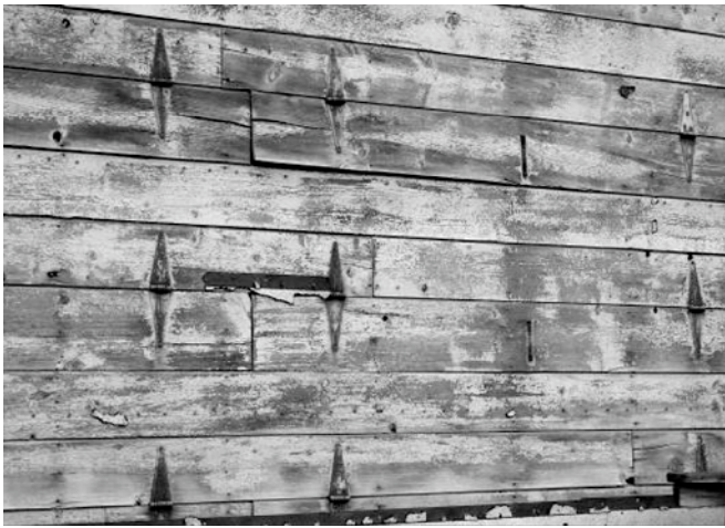
Detail of the barns' hinged horizontal siding.
