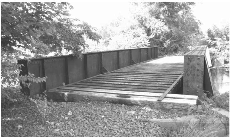
Plate-girder bridge, 1914, Boston Bridge Works, one of two ca. 1900 girder bridges on this two-mile section of the former Canal Line.
