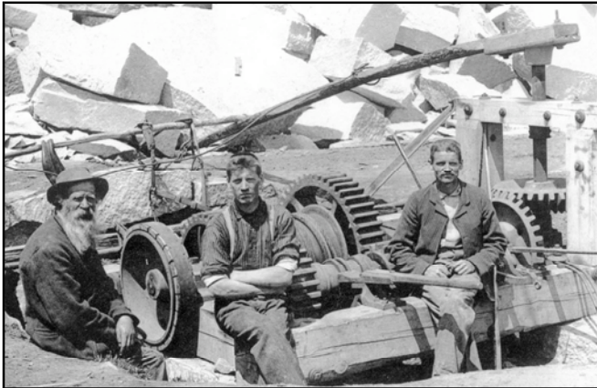
Figure 1. Horse Sweep-Powered Derrick Hoist, Barre, VT.
