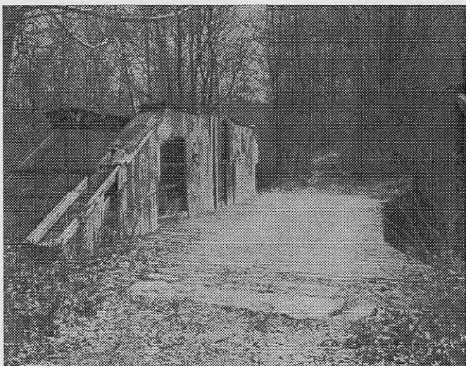
Fig. 4 Rollins Farm bridge spanning the Boston & Maine (now Guilford) RR main line at Rollinsford, NH, is a timber housed-pony-truss structure. It is unique among its handful of fellow survivors in being the last overhead railroad boxed pony now- standing, as well as for having three trusses in place, the third one (seen on the far left) to accomodate a cattle run.
