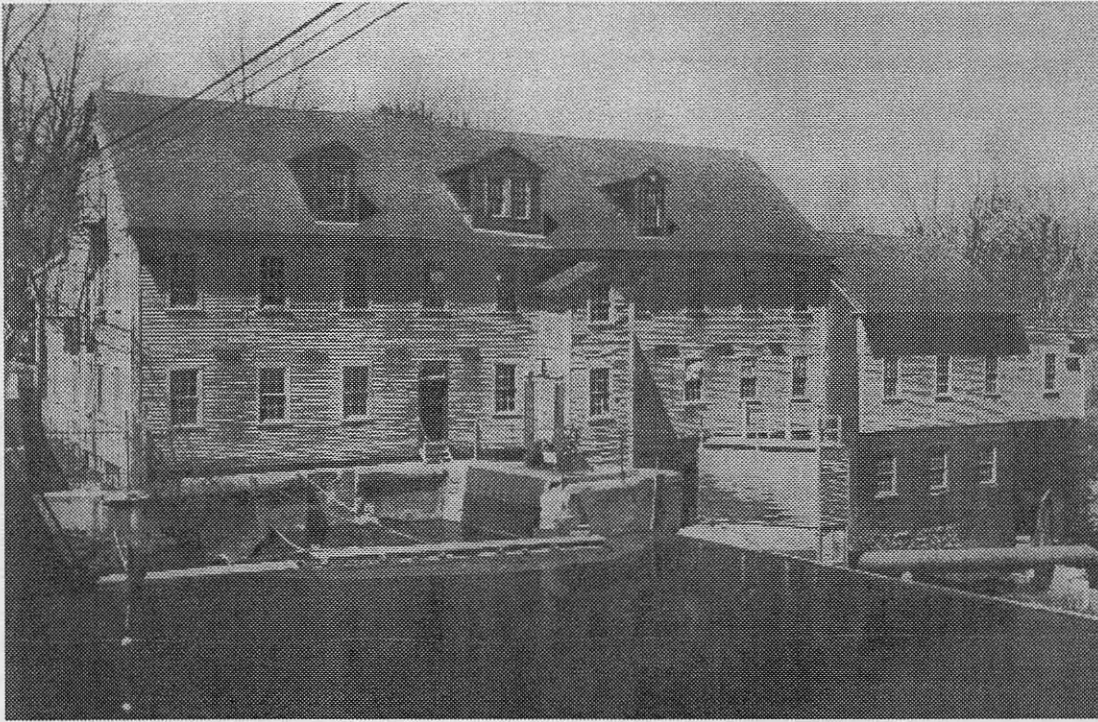
Fig. 3 The Burleigh woolen mill was constructed during the 1850s at Rocky Gorge, South Berwick, ME, using the falls of the Great Works or Aspenbedic River for the essential waterpower. The main mill building shown is a unique clapboard-over-brick construction. The Great Works mill site is one of the oldest in Maine, in use since the mid- 17th century.
