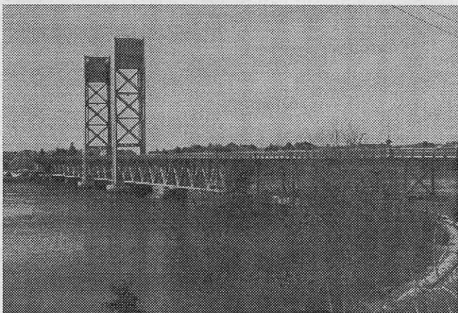
Fig. 1. The Sarah Mildred Long bridge, a vertical-lift structure completed in November 1940, spans the Piscataqua River between Portsmouth, NH, and Kittery, ME. Its lower deck accommodates the Boston & Maine (now Guilford) Railroad line curving downriver to serve the Portsmouth Naval Shipyard in
