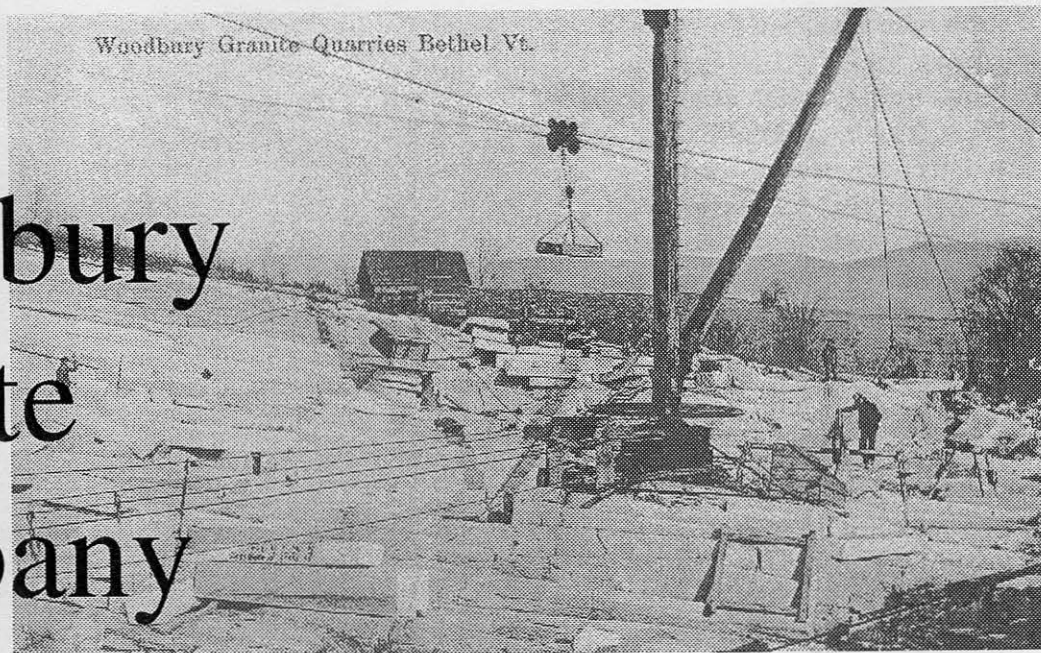
WGC Bethel Quarry Showing Blondin, Boom Derrick and Quarry Drill.
