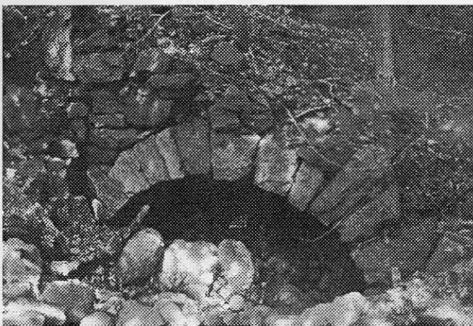
Stone-arched bridge, approximately six feet in span, across a former head race leading to the 1853 Charles Brockett carriage-spring factory site.
