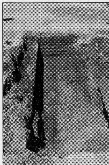
Above: T-rail used as concrete reinforcement in floor of ca. 1905 repair pit.
