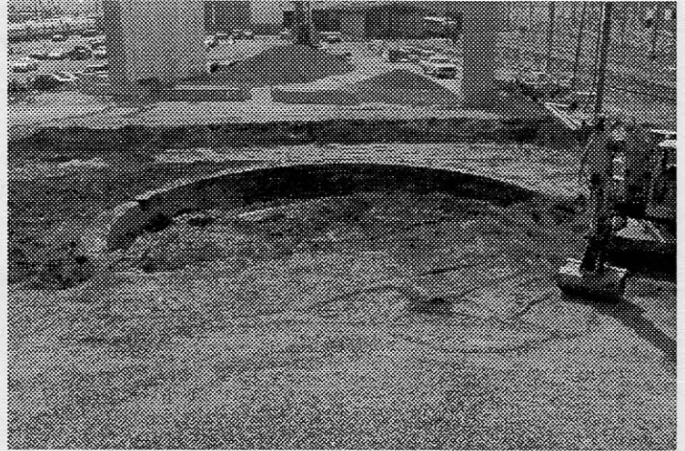
Portion of retaining wall for turntable pit, New Haven rail yard roundhouse, 1870. Piers in background are for the Church Street overpass.
