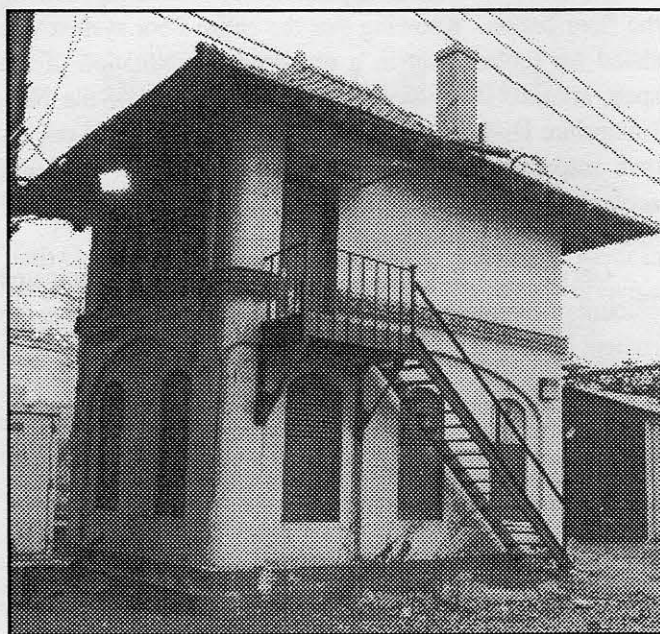
Photo 2. Looking northeast toward south and west facades. Note round-arched windows on first floor, set within arched, recessed surface.
