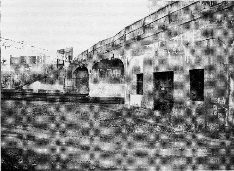
Photo 3. Window and door openings on north elevation of west pier. East abutment and wingwall in back-ground. Note standard high board fence along upper portion of bridge deck supported by metal stanchions.
