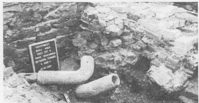
Photo 3. Discarded cast iron pipe sections that originally led to the tuyere air nozzle through the side of a bloomery forge. Also visible is the west exterior brickwork of the bloomery forge.
