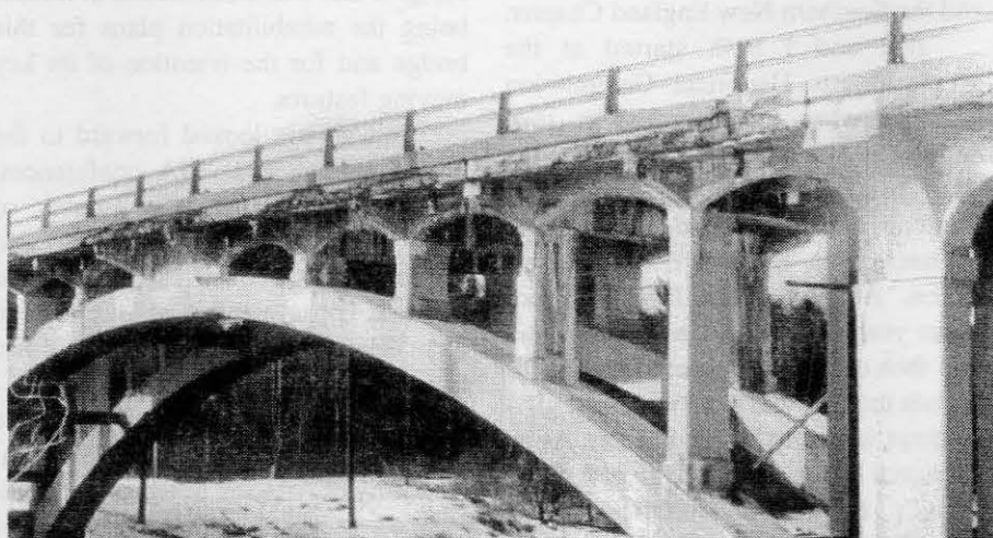
Plate 2 (above). The Kellyville bridge as it appeared shortly before demolition. The deterioration of the roadway is evident. Author's photo.
