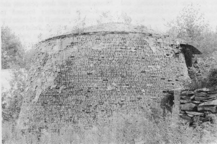
The brick 36-foot diameter Howard Family charcoal kiln (c. 1935) in Leverett, Massachusetts.
