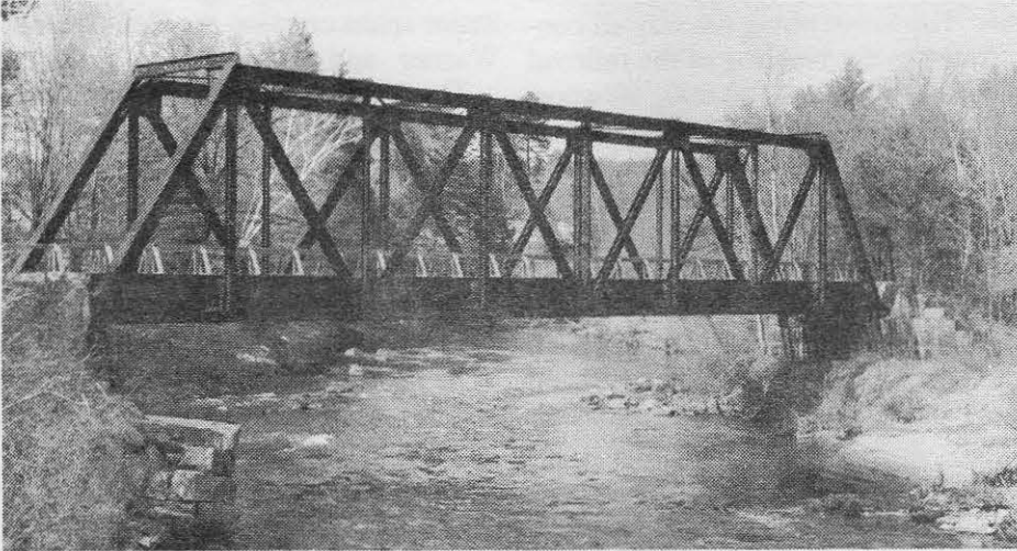
Bridge number 166, a 144 foot-long Warren truss which replaced Sibley's Bridge.
