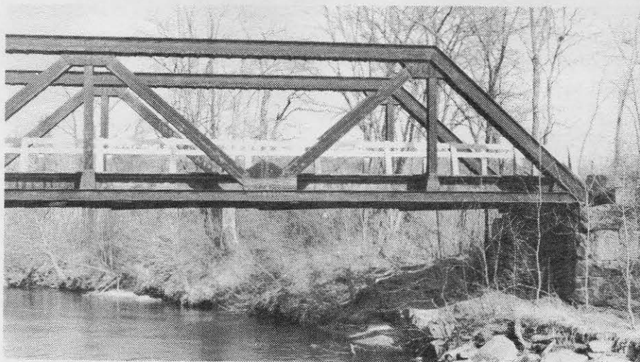
Bridge number 165, a 84 foot-long Warren truss with vertical tension members.
