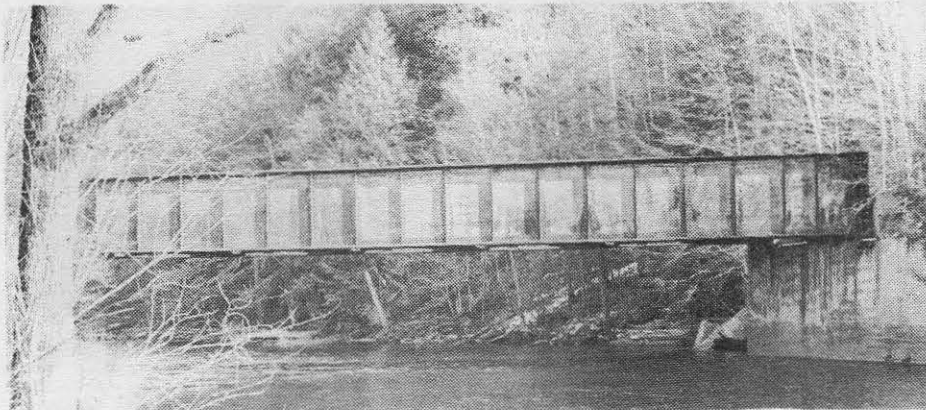
Bridge number 169, a 90 foot-long riveted plate girder truss.
