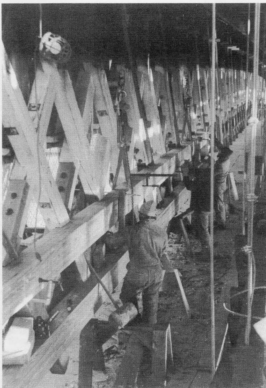
Installing the gluelams on the Town lattice.
