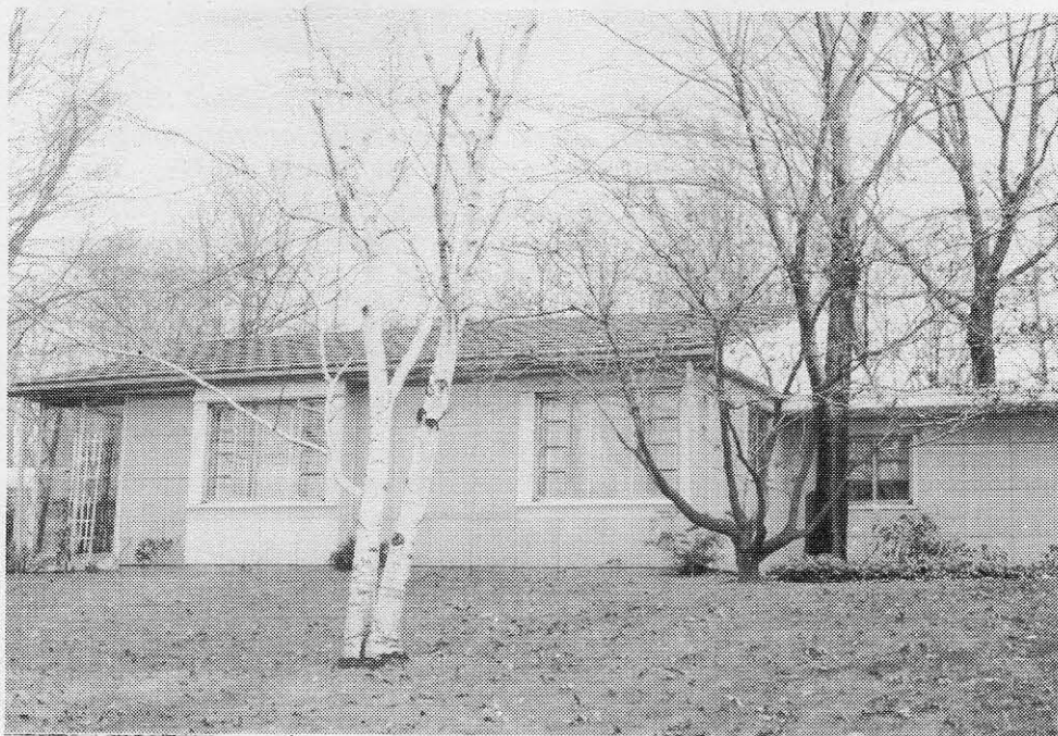
A Lustron prefab steel house.
