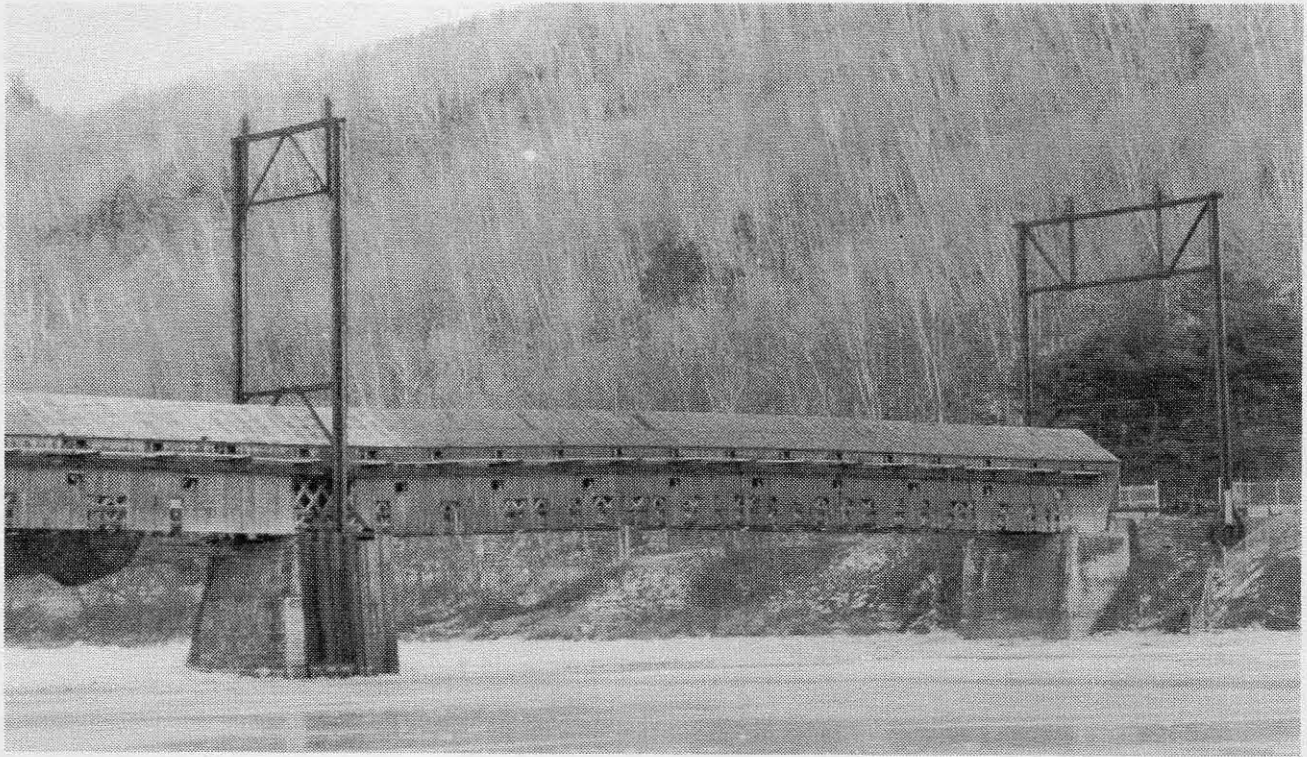
The eastern span of the Cornish-Windsor bridge with its suspension system rigged on temporary towers forcing a positive camber. The suspension wires connected to the needle beams supporting the upper chords cannot be seen in this photo.
