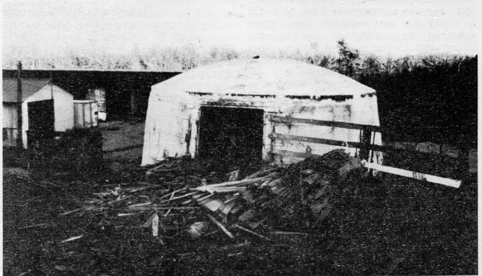
Upper loading door of one of the charcoal kilns in the process of charging with slabwood. Five kilns at Union are built against a similar embankment; two others are stand-alone (no embankment; loaded by lift truck and ladder).
